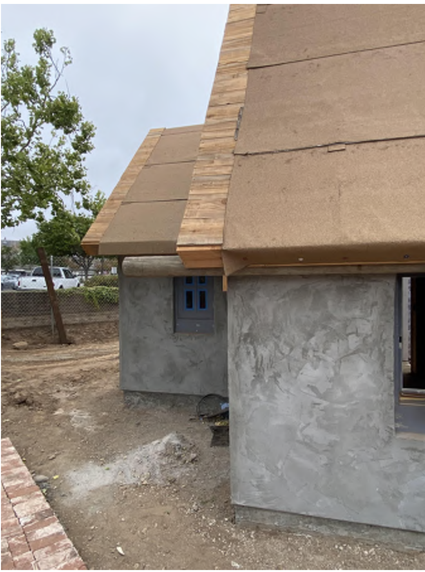
COTTAGE 4D AS-BUILT EAVE BEAM TAIL DETAIL
