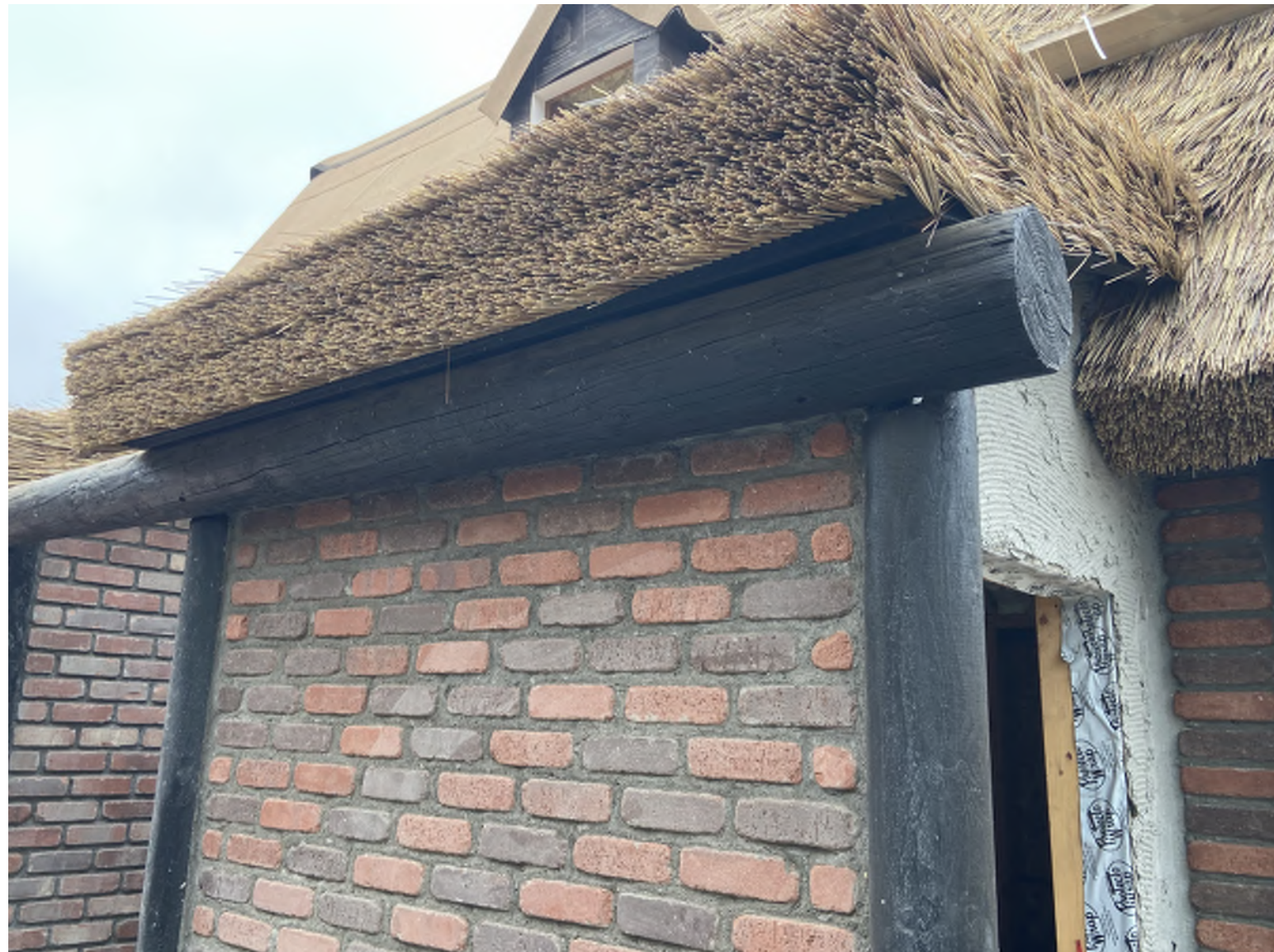
COTTAGE 8C AS-BUILT EAVE & ROOF DETAIL
