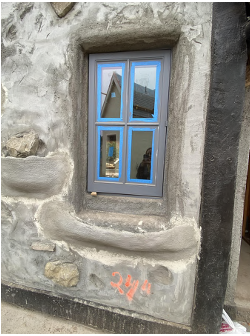
COTTAGE 6C AS-BUILT FRONT ELEVATION WINDOW DETAIL
