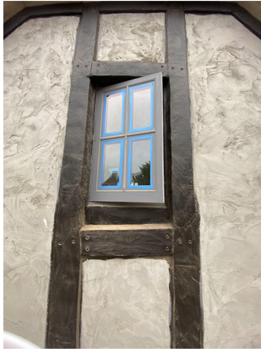
COTTAGE 3B AS-BUILT WINDOW & HALF TIMBER DETAIL
