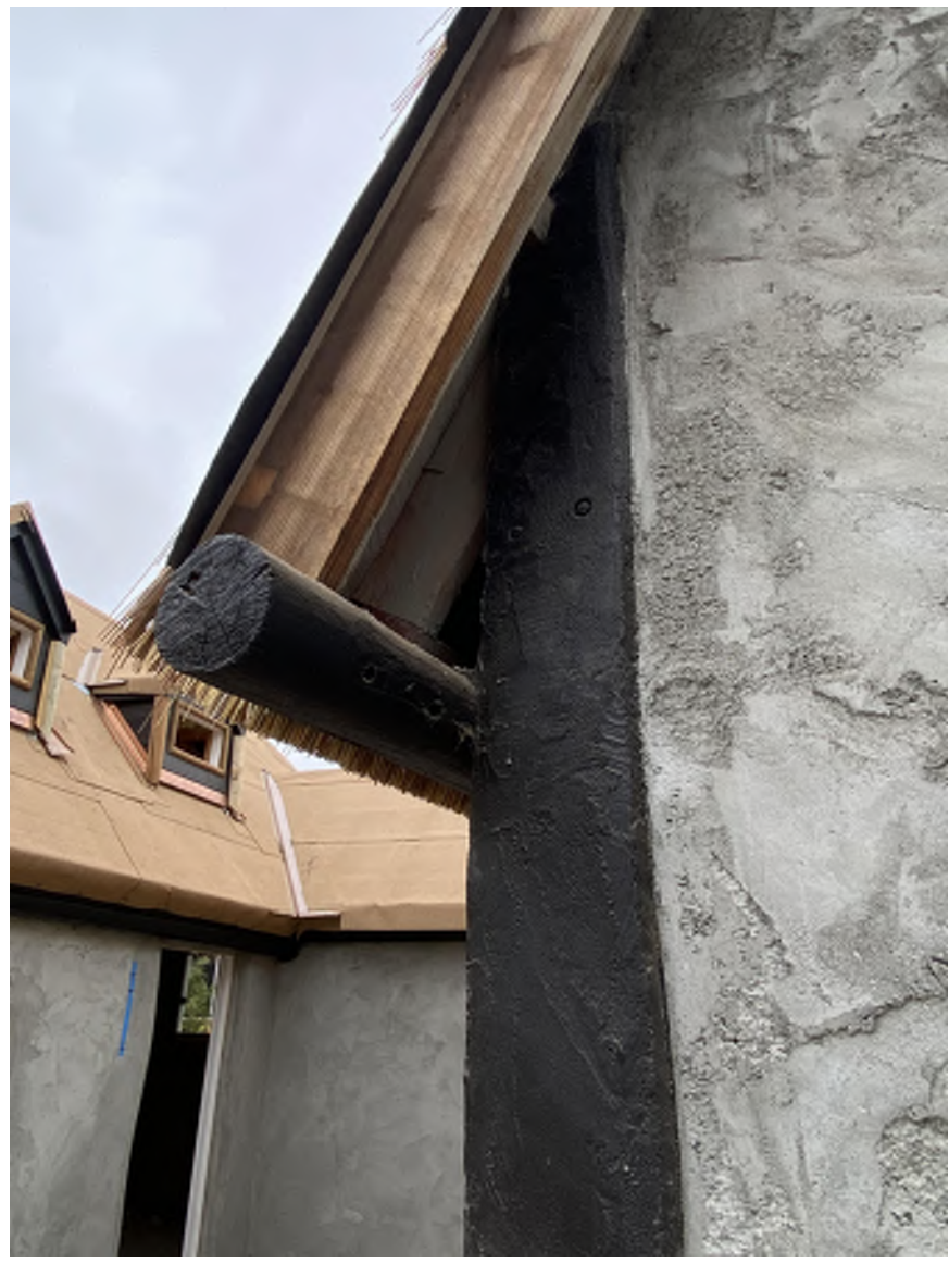
COTTAGE 6C AS-BUILT EAVE BEAM TAIL DETAIL
